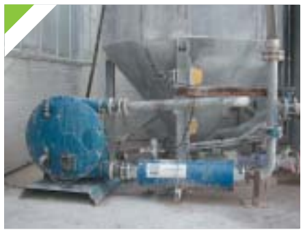
DL pump for titanium dioxide slurry transfer
