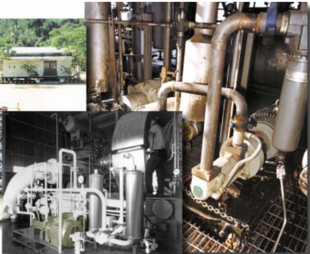
Sealless Mag drive 6D-156 pump on turbo expander gas sealing service
