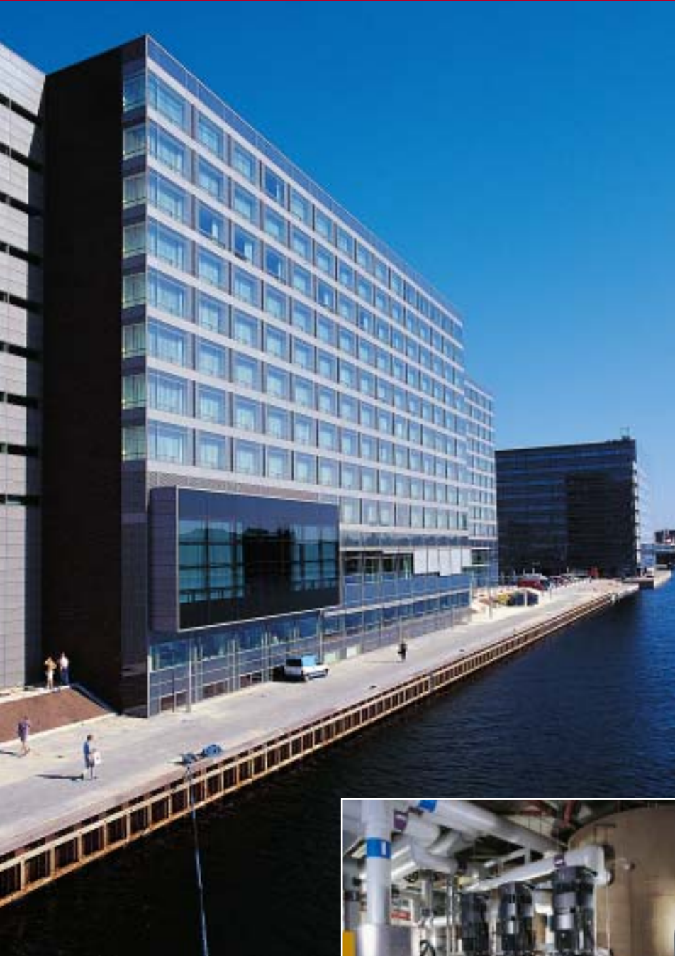
Grundfos Hydro 2000 booster installed at the Marriott Hotel, Copenhagen, Denmark, where it provides outstanding comfort and reliability regardless of variations in consumption.
