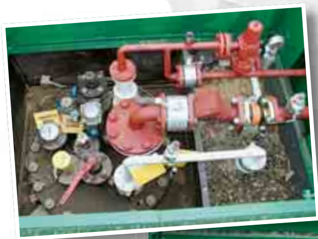
Underground autogas installation with one tank. Corken's autogas series pump replaced a previously installed submersible design.
