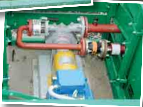
Underground autogas installation with one tank. Corken's autogas series pump replaced a previously installed submersible design.
