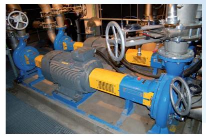
**Energy recovery in the paper industry** Pressurized and air-saturated waste water is pressure-relieved in the feed pipe to a micro-flotation plant. The energy recovered assists directly in driving a pump.
