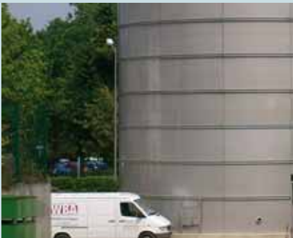
Wastewater Equalization Tank Diameter: 10.19 m Height: 10.50 m
