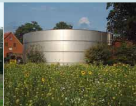
Manure Storage Tank Diameter: 15.75 m Height: 6.00 m
