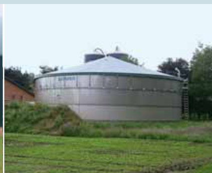
Agricultural Tank with Cover Diameter: 17.60 m Height: 6.00 m
