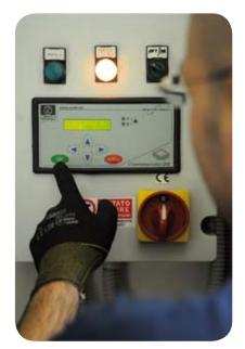
COMMANDER manages the operation of the pumps in a completely safe manner and allows maintenance interventions to be optimized thanks to the constant monitoring of the plant's key data.
