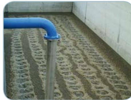
The Zenit range includes both disc and tube membrane air diffusers. Both models are fitted with high-quality membranes with perforation ensuring high oxygen transfer with low headloss, minimizing the relative energy consumption. Disc diffusers can be fitted with ball check valves. Zenit is able to design the most efficient aeration system for the customer's specifications, and supply the complete system, including detailed assembly drawings.
