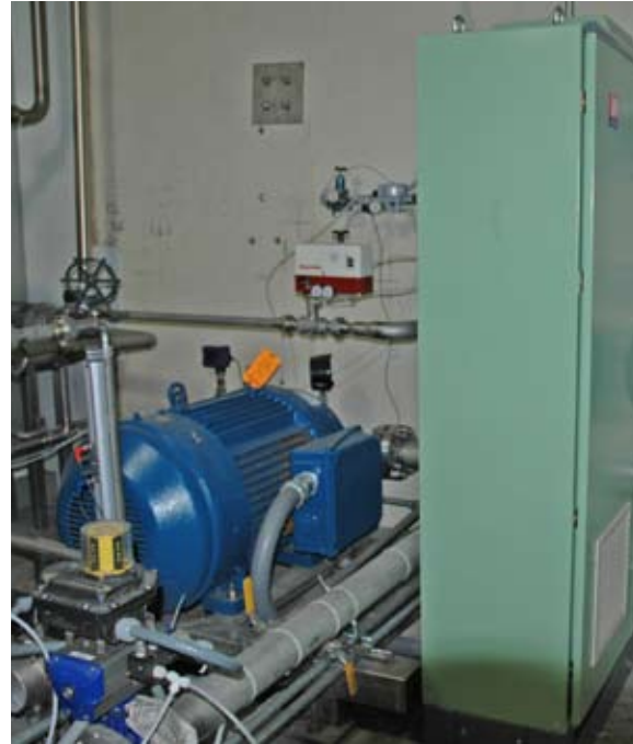
Roto-Jet VSR® & Converter In Service
