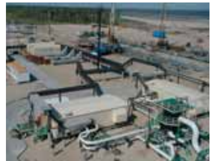
Phased installation: two MPP sets installed.
