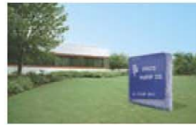
Price® Pump Co. manufacturing facility in Sonoma, CA.
