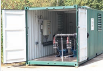
Stand-alone pumping station
