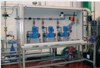
ChemSkid™ for ferric chloride injection
