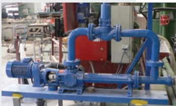
An industrial application featuring EcoMoineau with a bypass
