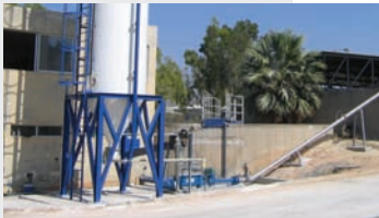
Lime treatment using Gavo™ in a sewage treatment plant
