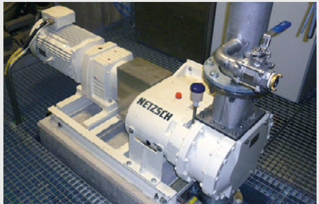
A TORNADO® pump in a paper factory for unloading Kaolin from tankers. Flow rate is 75 m 3 /h and pressure is 4 bar.
