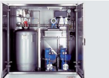
Flow proportional: precisely controlled odourant addition e. g. in the natural gas supply
