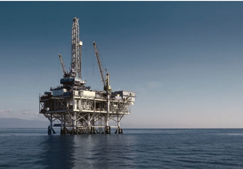
A typical installation of LEWA ecosmart pumps: Upstream processes in the oil & gas industry.
