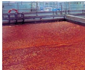
The next step for this sludge produced by a Clari-DAF system is dewatering equipment.
