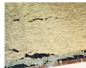
The floating sludge blanket—a mass of solids formed by the microbubbles that have captured and floated the pin floc to the surface—is easily removed with a mechanical skimmer or by hydraulic overflow.
