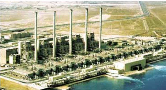
Jebel Ali Gas Turbine & Desalination Station "E"
