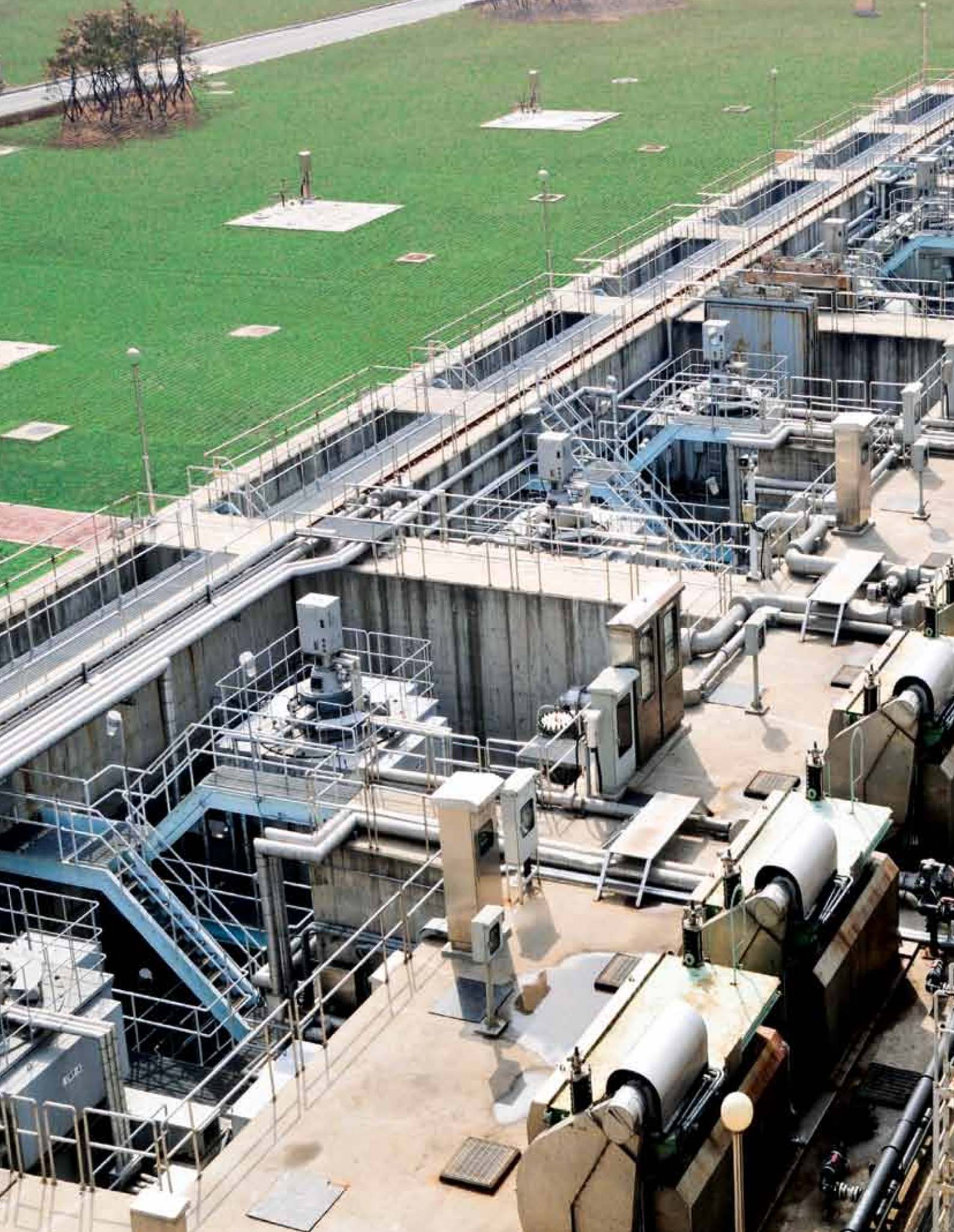
Circulating Water Pump for Yonghung Thermal Power Plant, Units 1 & 2, KOREA (1100m 3 /min X 20m X 4600kW, Model 3000VKANM, Variable pitch vane type)
