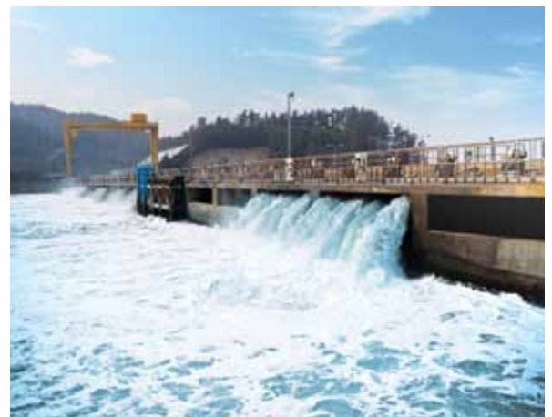
Seawater Lift Pump for Taeon Thermal Power Plant
