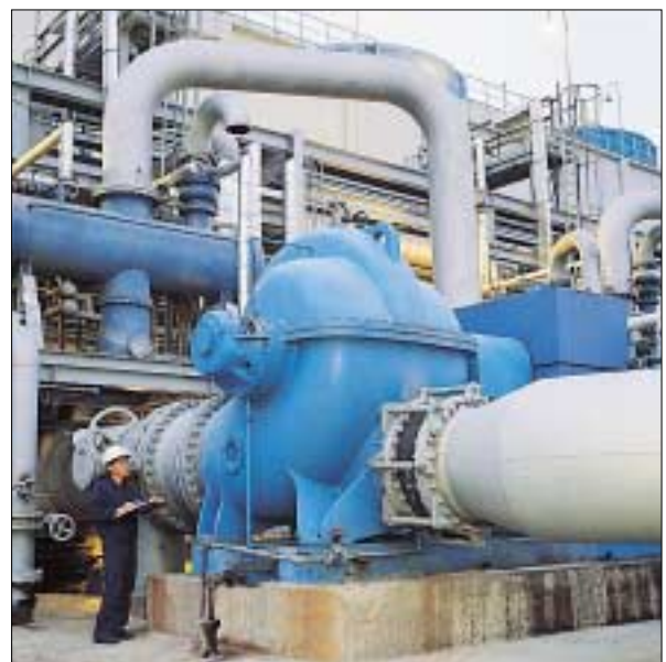
Cooling water pump of Hyundai Petrochemical Co., Ltd., Korea (Model 1050 × 750HDM, HDGT)
