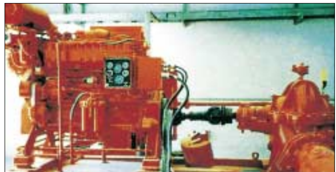
Engine driven fire fighting pump for Jebel Ali Desalination plant, Dubai, U.A.E. (Model 300 × 250HDE)
