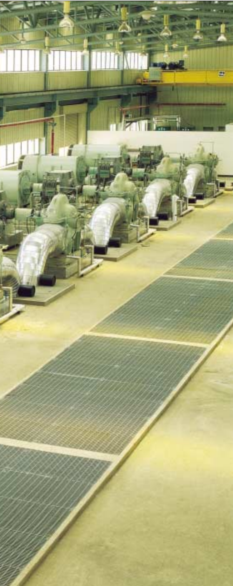
▲ District heating water supply pumps for Bun-Dang, Korea (Model 600 × 400HDM)
