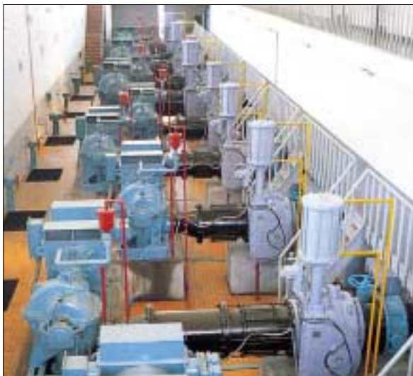
City water supply pumps, Dae-Gu, Korea (Bottom suction, Model 400 × 300HDM)
