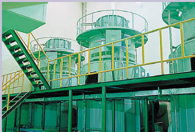
De-watering Pump for Dockyard 1500VKM
