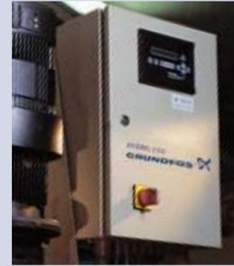
The CRE pumps used for the booster systems are equipped with Grundfos' own frequency converter-controlled motors and thus provide the ultimate in pumping technology available on the market today.
