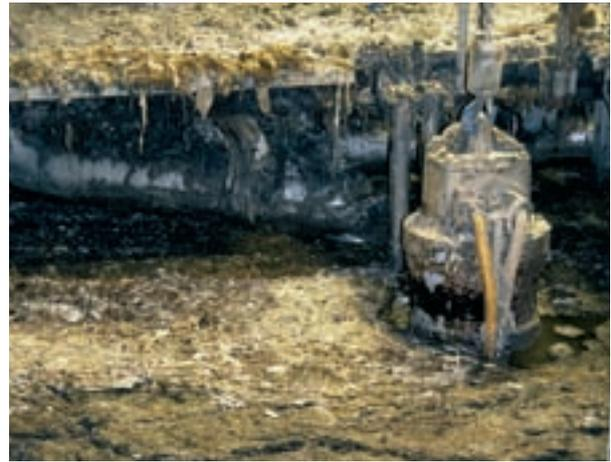
Flygt submersibles operate directly in the pumped liquid. This means low construction costs because Flygt pumps don't require a special housing or a superstructure. Operating submerged also means that our pumps take up very little space, are quiet and do not need extra cooling.
