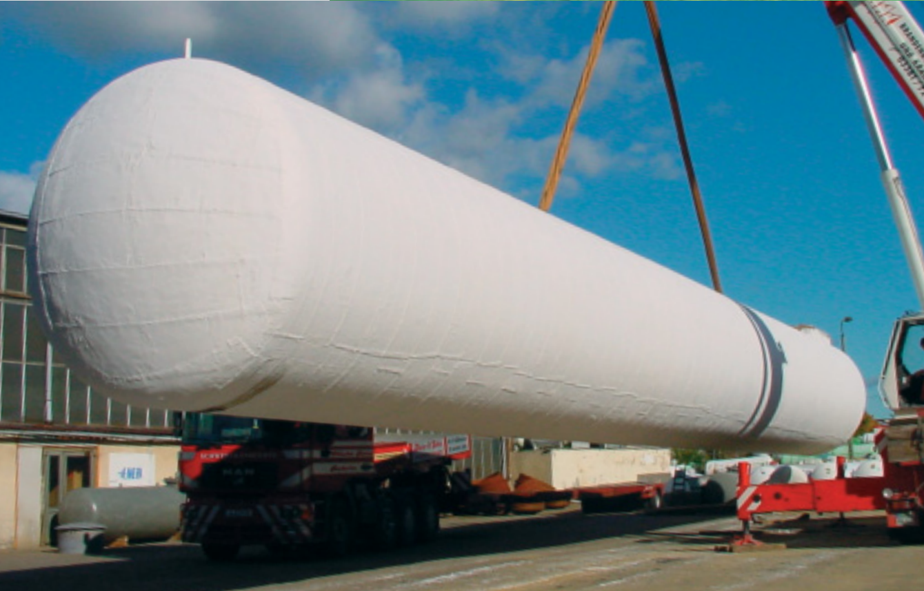
Overhauled custom tank with bitumen coating.
