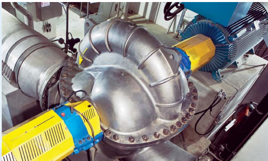
▲ Double suction split case pump for conveying water and suspensions
